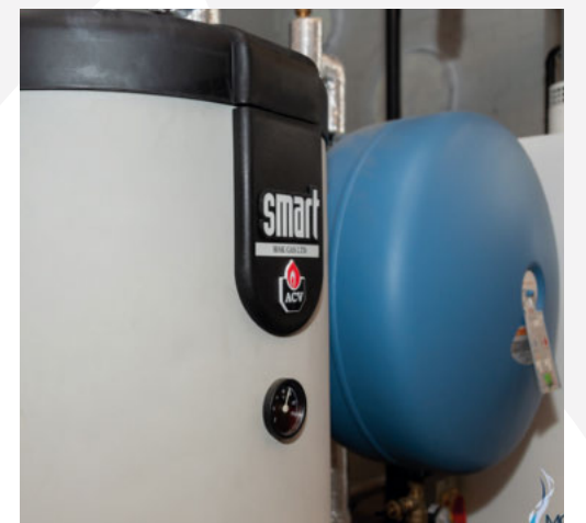
The Smart tank-in-tank cylinder provides quick recovery domestic hot water to meet the needs of the schools' bathrooms
